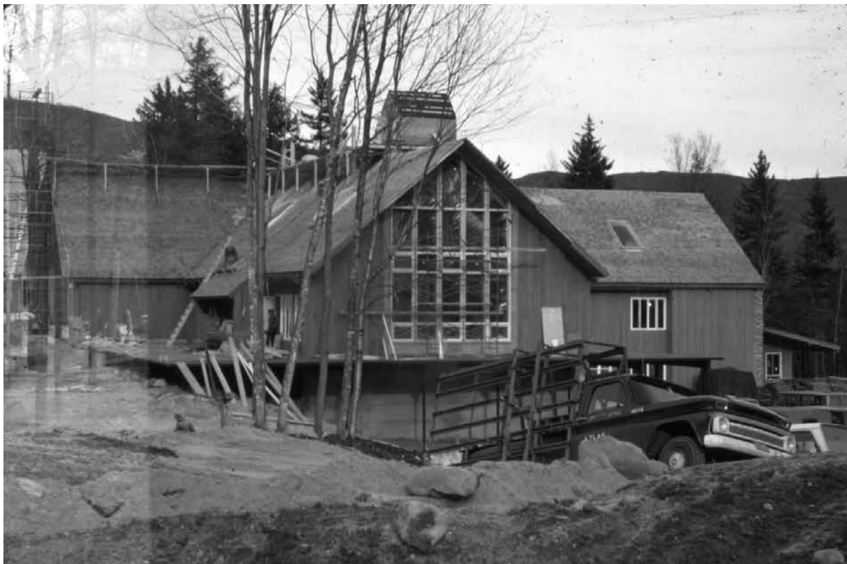
The Waterville Valley north complex base lodge under construction in the fall of 1966. The adjoining south complex housed the offices of the company.
