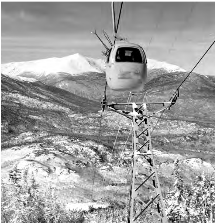
In the winter of 1958, the first gondola lift in the country began operating at Wildcat. The Carlevaro-Savio manufacturer was Italian, and the lift with its enclosed 2-person cabin was selected by the developers for its protection from the weather. The gondola operated until 1999.
