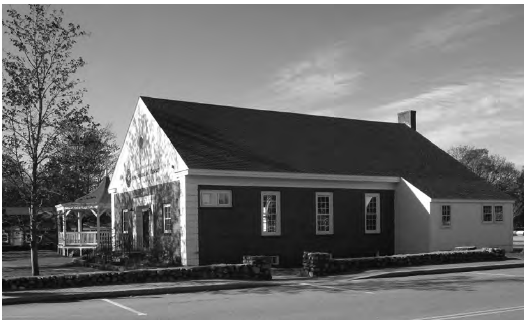
The former North Conway Community Center, seen here with its new roof, will soon host the Museum’s Eastern Slope Branch.
