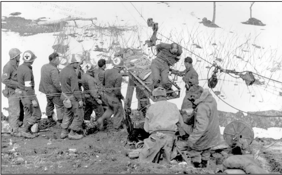
This portable tramway was erected by Company D of the 126th Mountain Engineers on February 21, just after the Riva Ridge action, to resupply troops still fighting off counterattacks on the ridge and to evacuate casualties, as seen here. The tramway was built on Mount Cappel Buso, one of the summits of Riva, and gained 602 vertical feet over a 2,000 foot distance. In the first day of operation, 50 casualties were evacuated, 30 of them wounded and the remainder killed in action. Five tons of ammunition and other supplies were ferried up the line. This was the first aerial tramway ever used in combat in the U.S. Army. Several weeks later, Company D erected a second tramway to connect two sides of Sprilla Road, cutting off a loop that extended into enemy territory, enabling a continuous supply route. Crossing a deep ravine, the tramway connected the towns of Castellaccio and Campidello and transported 200 wounded soldiers and tons of supplies from March 10 until April 2.
